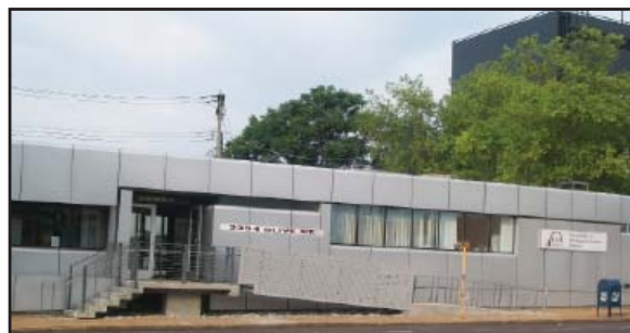
(Pictured at left) DD Resources' newly added ramp.
